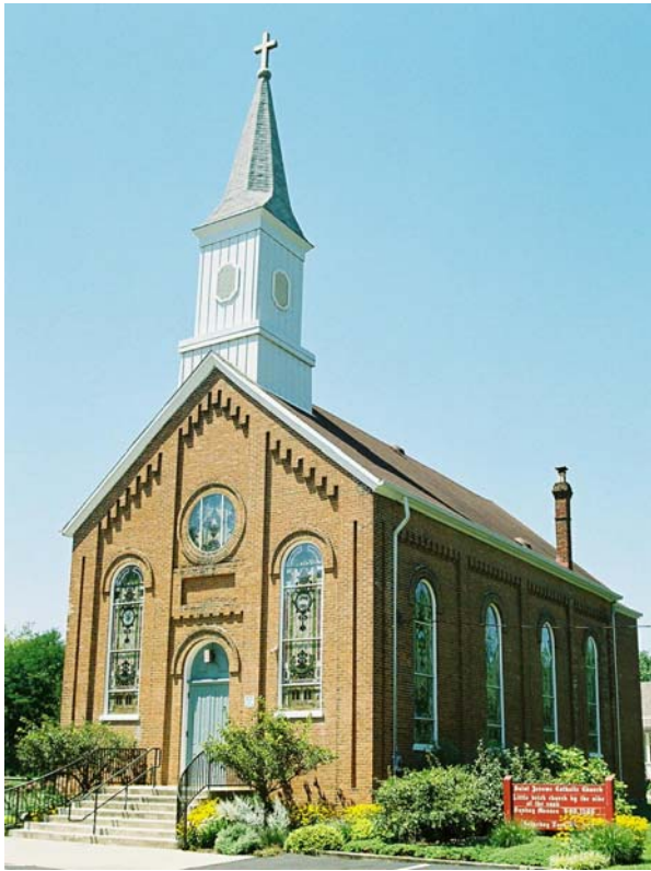
131 Rohde Street, California, Ohio
